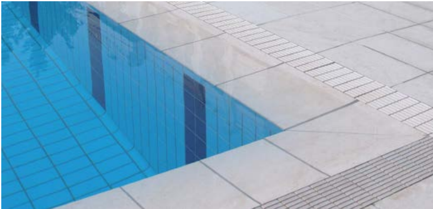
Rehabilitación de piscina comunitaria con borde 500 Beige Stone. Restoration of community pool with 500 Beige Stone border.
